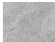
Bathroom Wall Tile
